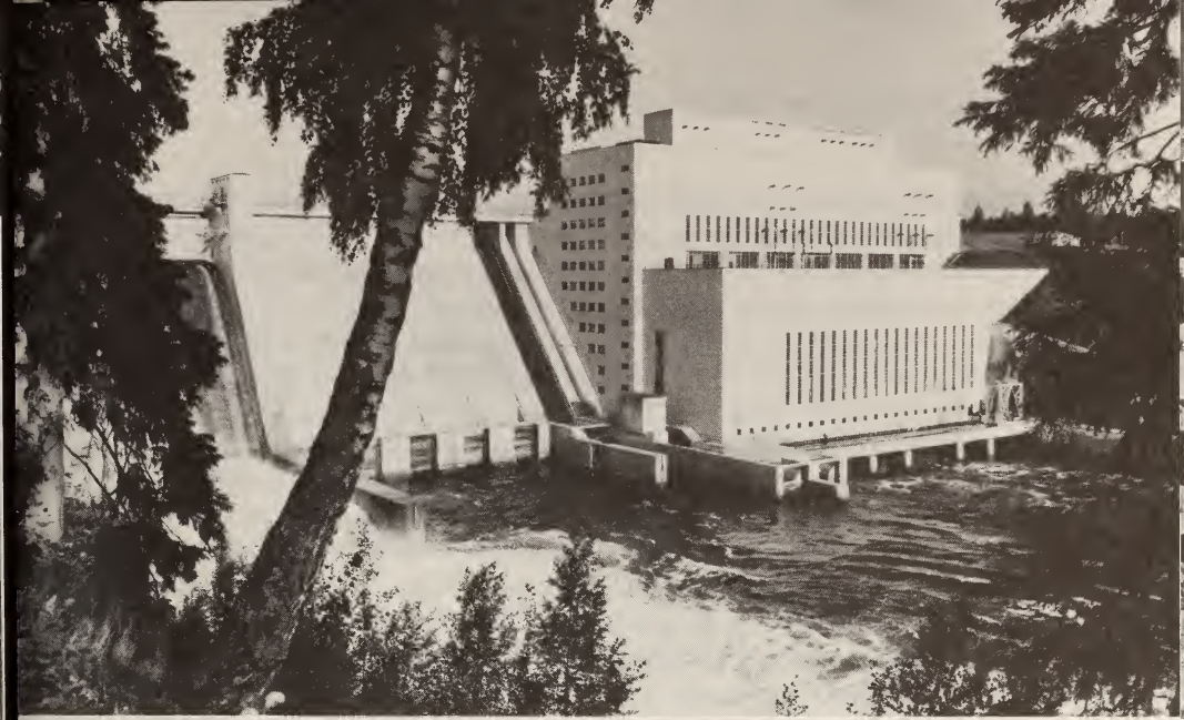
Pyhäkoski hydroelectric power plant, one of the largest of its kind in Finland, located about twenty-five kilometers east of Oulu Courtesy Embassy of Finland, Washington
